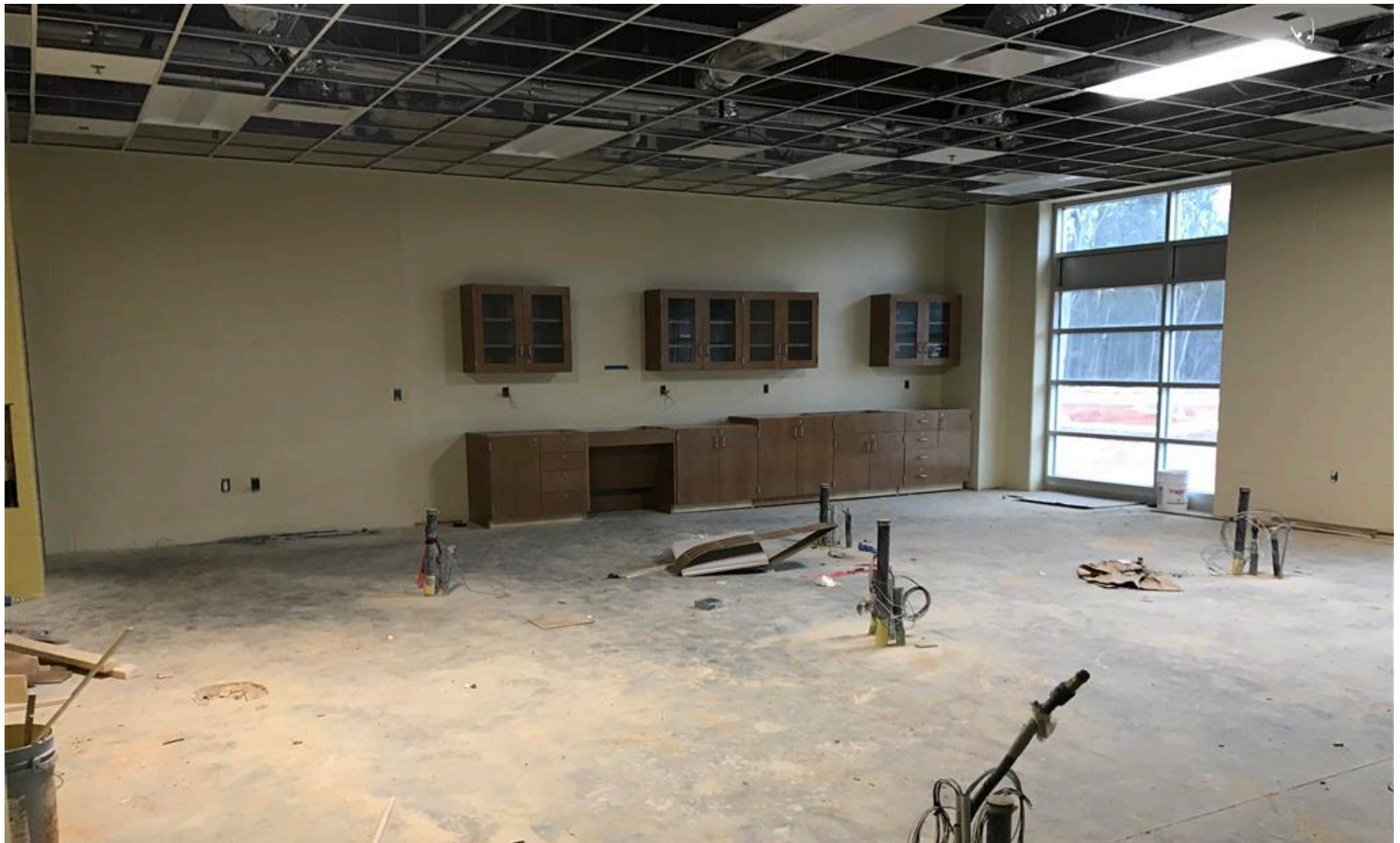
Ceilings, cabinets and counters being installed in classrooms.
