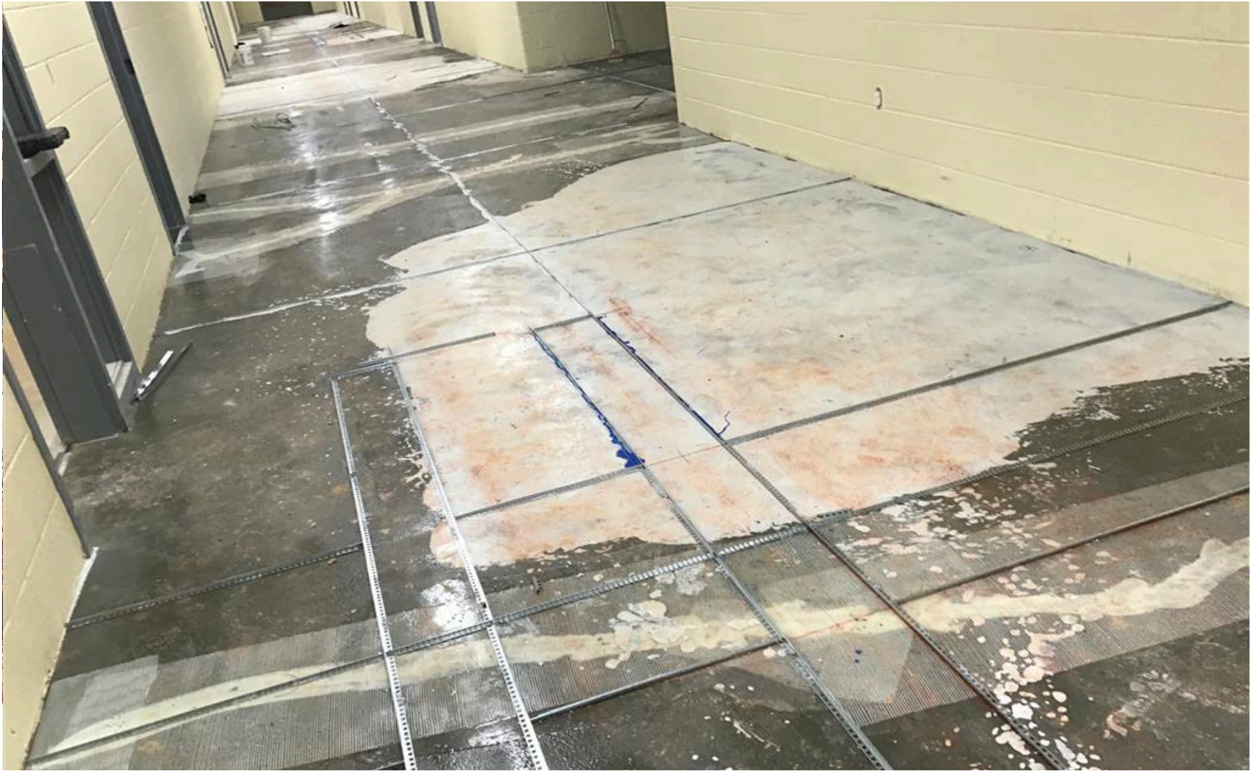
Terrazzo flooring being installed.
